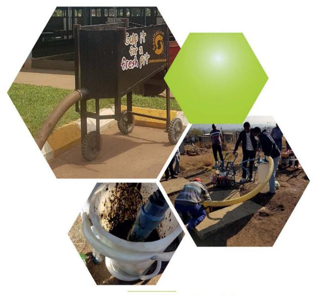
▲ Figure 4 : Semi-mechanized pit emptying
