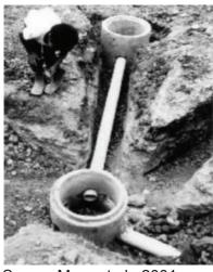
Source:Mara et al., 2001 Figure 8.7 Junction chamber for simplified sewerage using larger diameter concrete pipes, used in Guatemala
