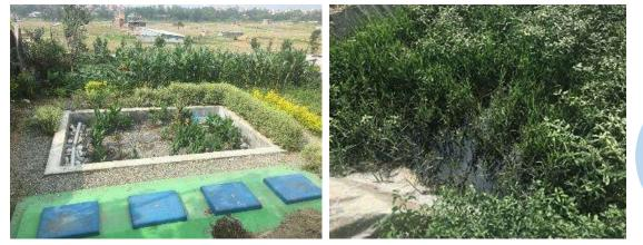
ABR, Constructed Wetland and Policing Pond for wastewater treatment
