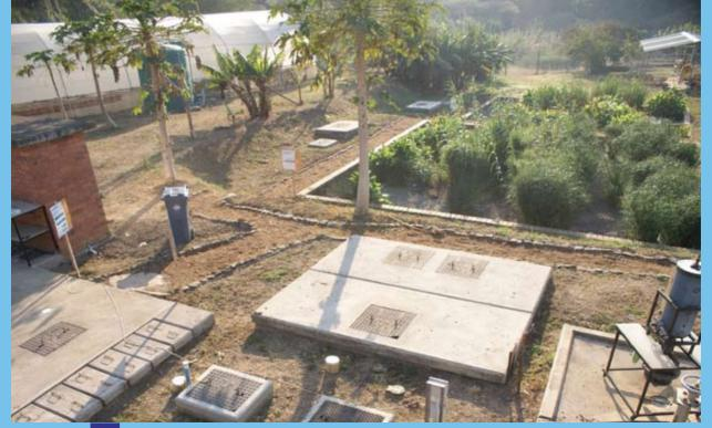
*Horizontal Planted Gravel Filter* - The Horizontal Planted Gravel Filter provides additional treatment as the wastewater flows horizontally through the planted gravel bed. Organics are further degraded, and more nutrients and pathogens are removed.
