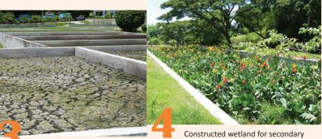
Sand drying beds with underdrains
