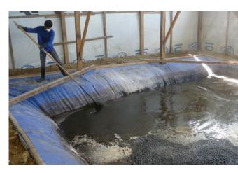
Figure 26. This is a reactor pit in Palo, Leyte, which was first built after Super Typhoon Yolanda. Here, workers stabilize the septage with lime, then transfer it to sand drying beds.
