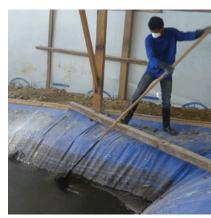
Figure 22. Hand mixing is inefficient and labor intensive. Mechanical mixing with paddles, blowers or pumps is better.
