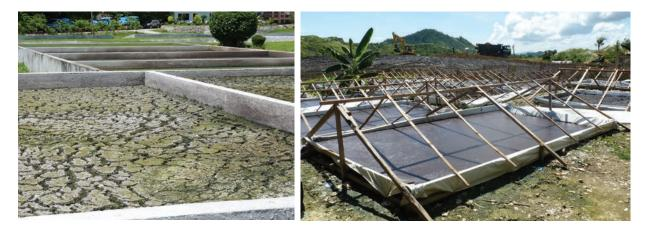
Figures 10 and 11. Sand drying beds (left) showing characteristic "cracks" on the sludge surface, indicating sludge is sufficiently dewatered to transfer to bulk biosolids storage area (about 25% dry solids). Sludge drying beds (right) with canvas tents (removed) to shed stormwater which allows dewatering even during rainy season.
