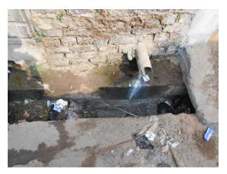
Figure 9: Outlet of a containment unit drains directly into a drain
