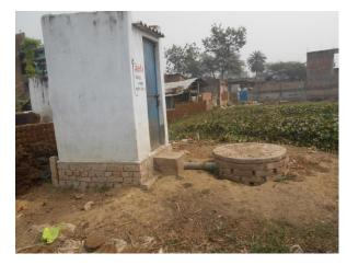
78% of the Rectangular containment units' resembled septic tanks in the construction and had elements such as baffle wall, these tanks were common across the clusters as they had huge storage volumes, which were indeed preferred by the household. The sizes of these tanks varied between 2 - 57 M<sup>3</sup>. In general the depth of these tanks varies between 3 - 15 feet. 78 % of these tanks claimed to be lined at the bottom, while 85 % of septic tanks claimed to have watertight walls.
