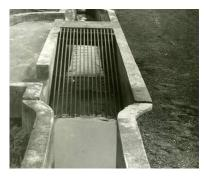
Grit chambers are like sedimentation tanks, designed to separate the intended
