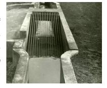
collected by manually scrapping the screen with a rake or similar arrangement. The collected trash will be stored and disposed along with municipal solid waste collection facility of the Bhagalpur municipality.
