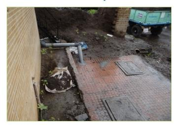
Toilets directly connected to drains
