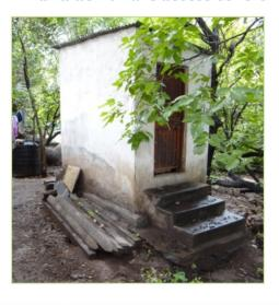
Inaccessible septic tanks with sealed tops
