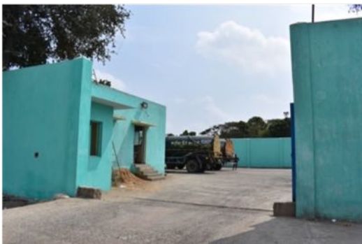
Entrance of the decanting station
